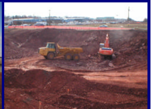
Grading at Route 625
