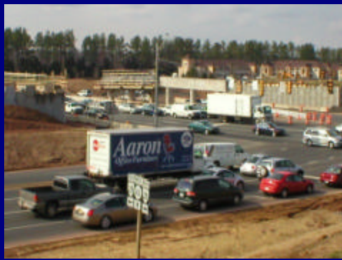
Substructure for the Route 606 Bridge over Route 28
