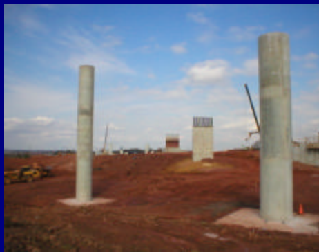
Support piers for future Flyover Bridge at Route 625.
